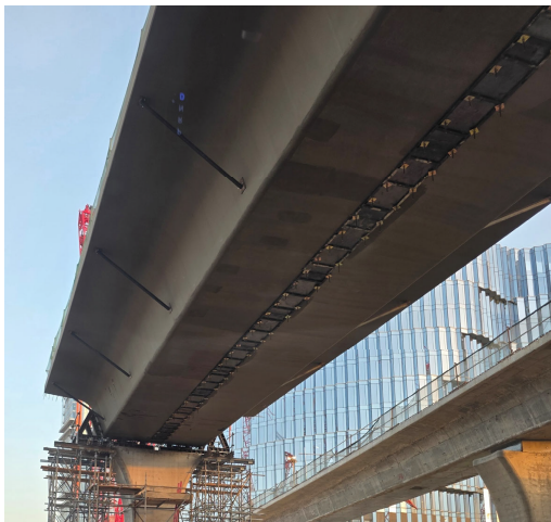
Figure 17. Bottom slab connection. Courtesy of e.construct.
